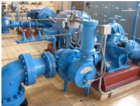
Pumps and Piping after stripping, priming, and repainting
