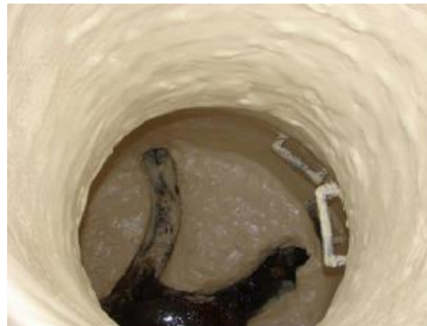
Coatings Applied to Manholes, Tanks, Pits, Wet Wells
