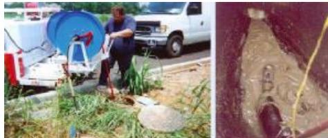
High pressure jetting is the most common method used to remove root infiltration growth within sewer lines that routinely cause blockages. High pressure water at 4,000 PSI with the proper nozzle cuts roots close to the pipe wall surface, then flushes the residue downstream.
