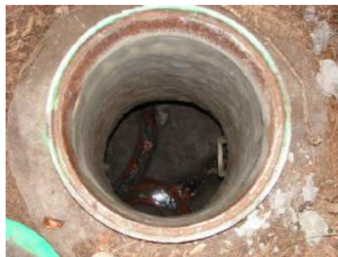
Man Hole after Mortar Repair
