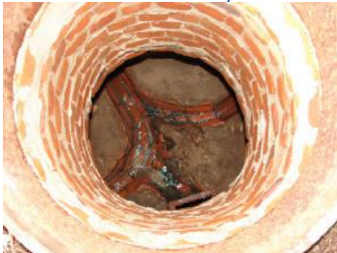
Man Hole after Initial Repair and Cleaning
