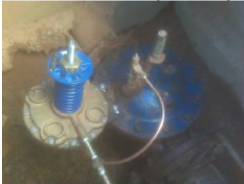
6 Inch Altitude valve rebuilt and pilot valve replaced
