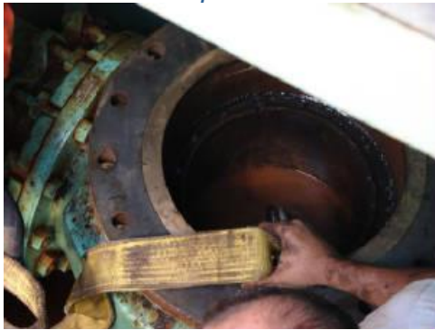
12 Inch Altitude Valve Piston being removed
