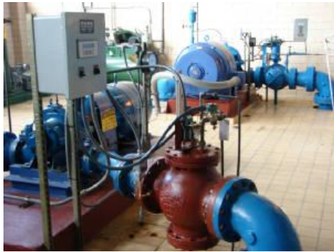
Replaced Control Valve
