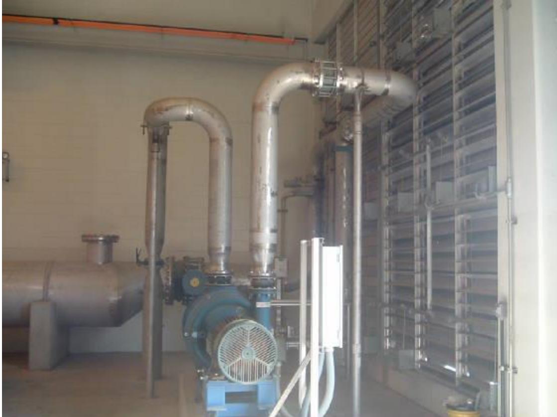
Blower and Stainless Steel Air Header Added
