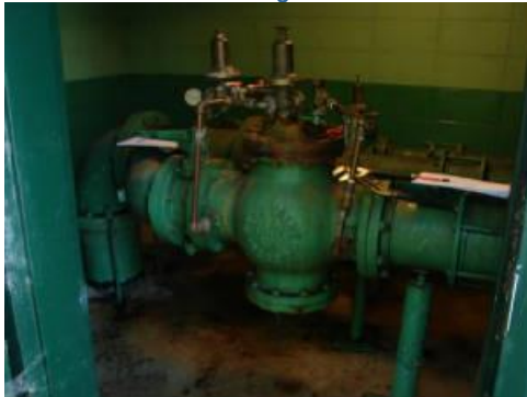
8 Inch Pressure Sustaining Valve and Pilots rebuilt
