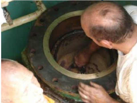
12 Inch Altitude Valve Piston being installed after rebuilding valve
