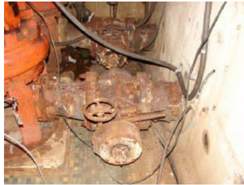
Valves Prior to Replacement in a Pump Station
