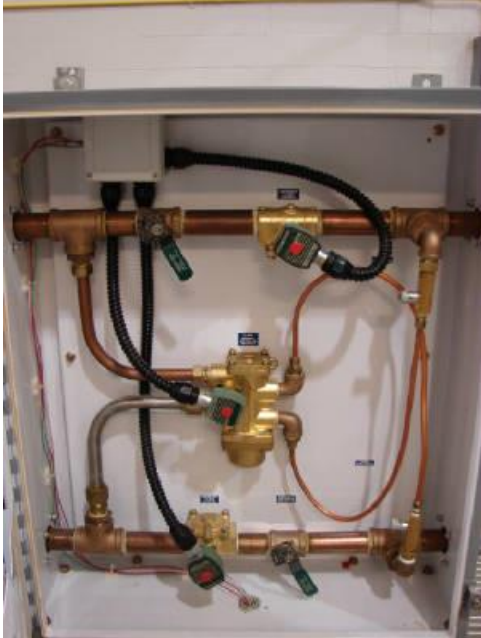
Pump Control Repair
