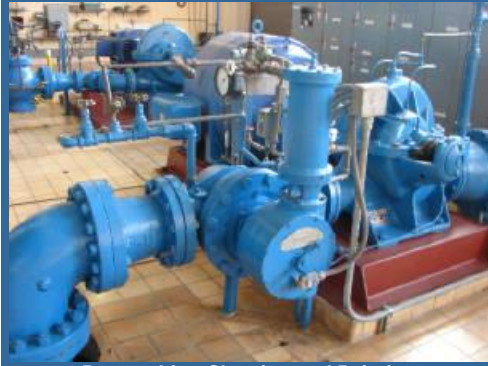
Pumps After Cleaning and Painting
