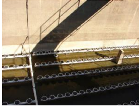
Aeration Header Repair and Replacement
