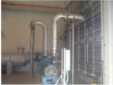
Blower and Stainless Steel Piping Installation
