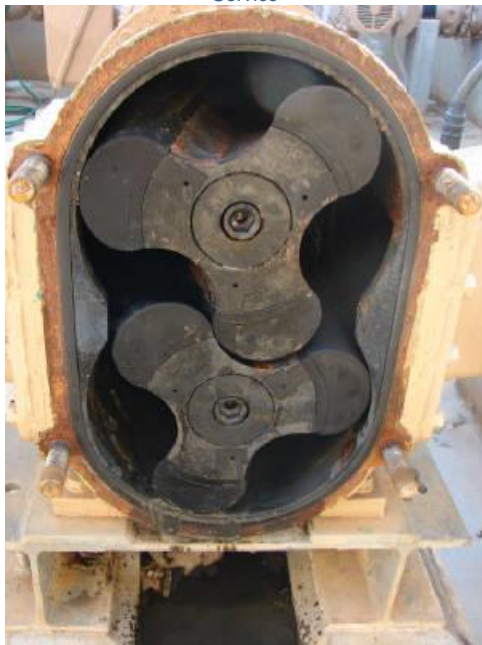
Replaced Pumps Seals, Checked Lobes for Wear, and Performed Preventive Maintenance
