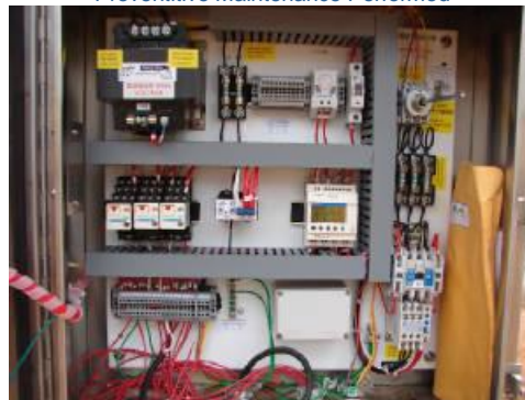
Control Panel and Ancillary Equipment Start Up
