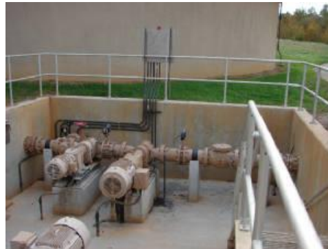
Pump Seals Replaced and Cutter Teeth on Shredder Preventive Maintenance Performed
