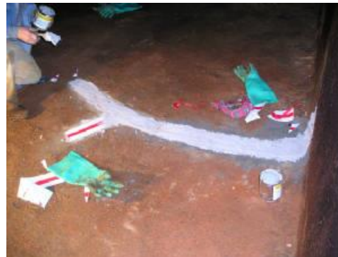
Repair Made to Bridge Crack and Cover with a Patch - No More Evidence of Water Loss
