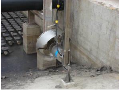
Mixer and Mast Installation, Including Stainless Steel Fabrication to Accomodate Mast
