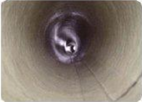
Pipe after Liner Installed
