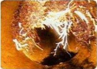
Pipe Prior to Root Removal and Lining
