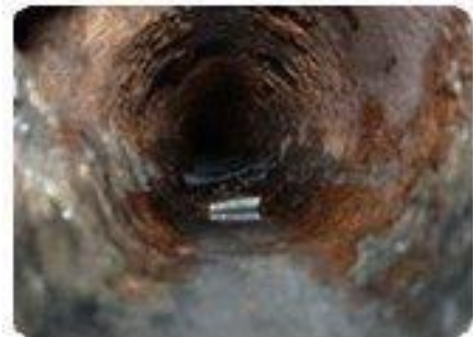
Pipe with Build Up Prior to Liner Installation
