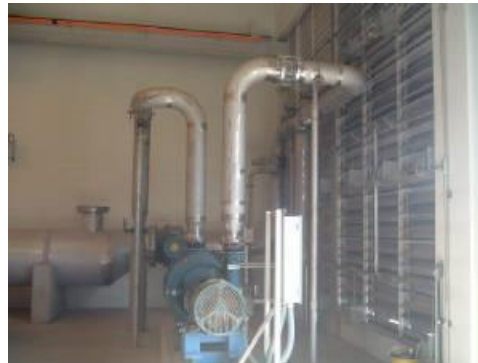
Fabrication of Stainless Steel Piping, and Valves
