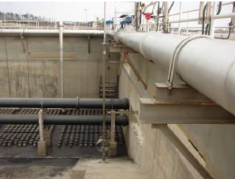
Mixer, Stainless Steel Shaft, and Stainless Fabrication Including Installation
