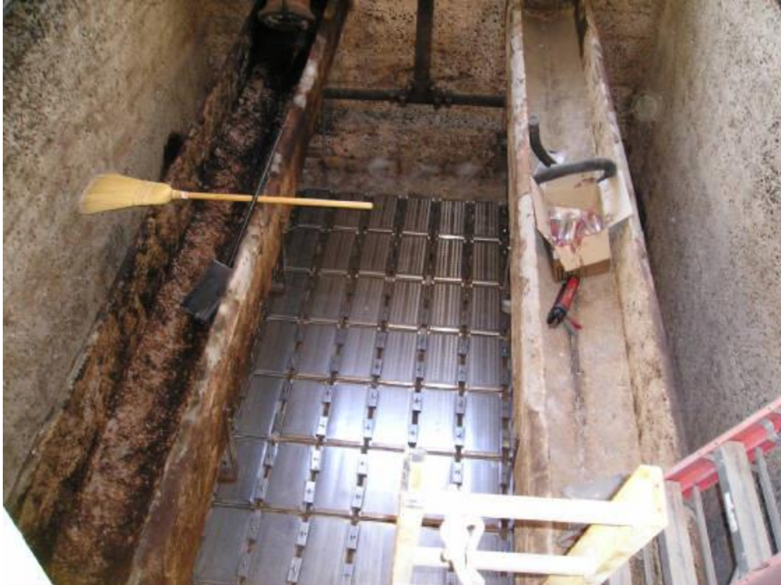
Adding New Stainless Bottoms to Filter
